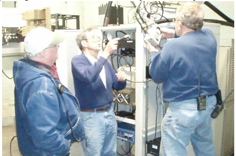
Tech Committee Members at work on the new repeaters.
