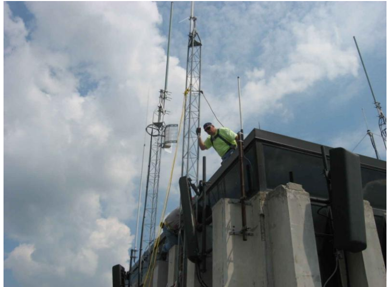
Steve, W8TER holds the new tower in place as Mark, KC8TVP secures it to the top mounting bracket. kb8fxj photo
