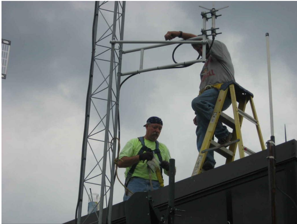
Steve, W8TER and Mark, KC8TVP attach the 440 antenna to a new sidearm.
